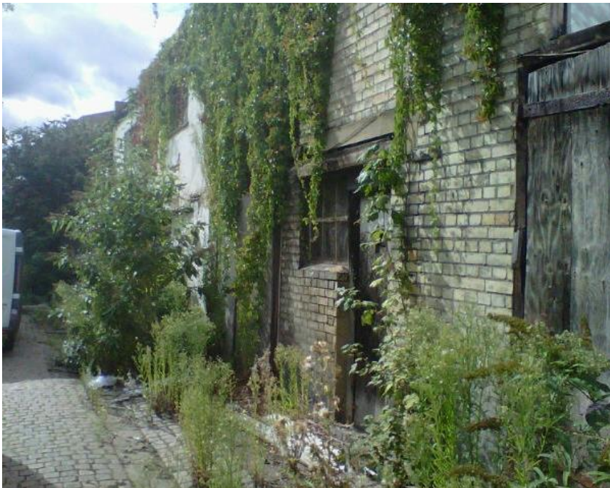
Image 1: View of existing derelict buildings at the site looking along the Mews in SE direction.
