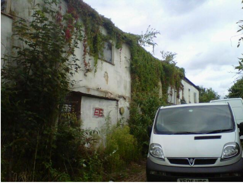
Image 2: Existing derelict buildings looking along the Mews in NE direction.
